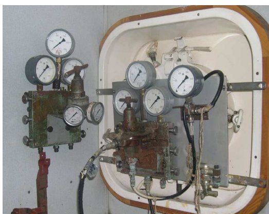
Figure 15: Air distribution panel..
